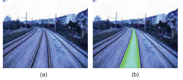
Fig. 7. Examples of railroad track extraction on various scenes: a) Original image b) Result of railroad track extraction
